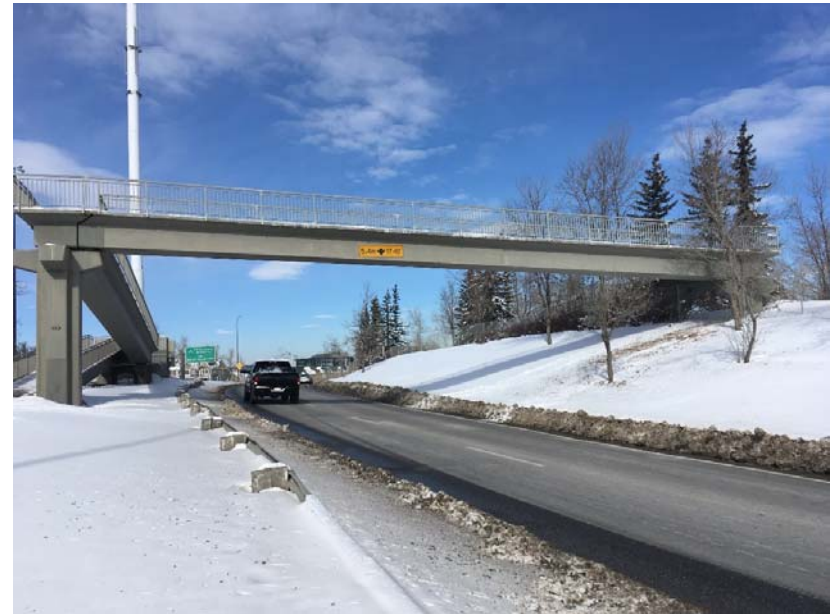
Example of Precast Box Girder Bridge in Calgary
